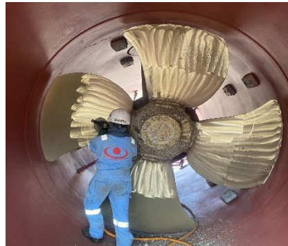
POLISHING OF PROPELLER
