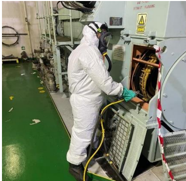
IN-SITU CHEMICAL CLEANING OF ALTERNATOR
